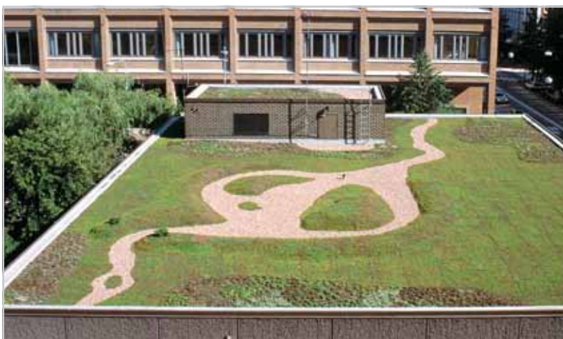
Veg Tech's moss-sedum roof vegetation
